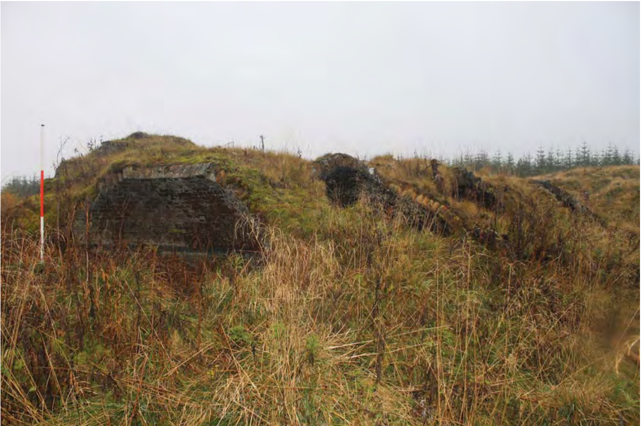
Plate 3: General view of the main coke ovens (F01) to the west side, taken from the west
