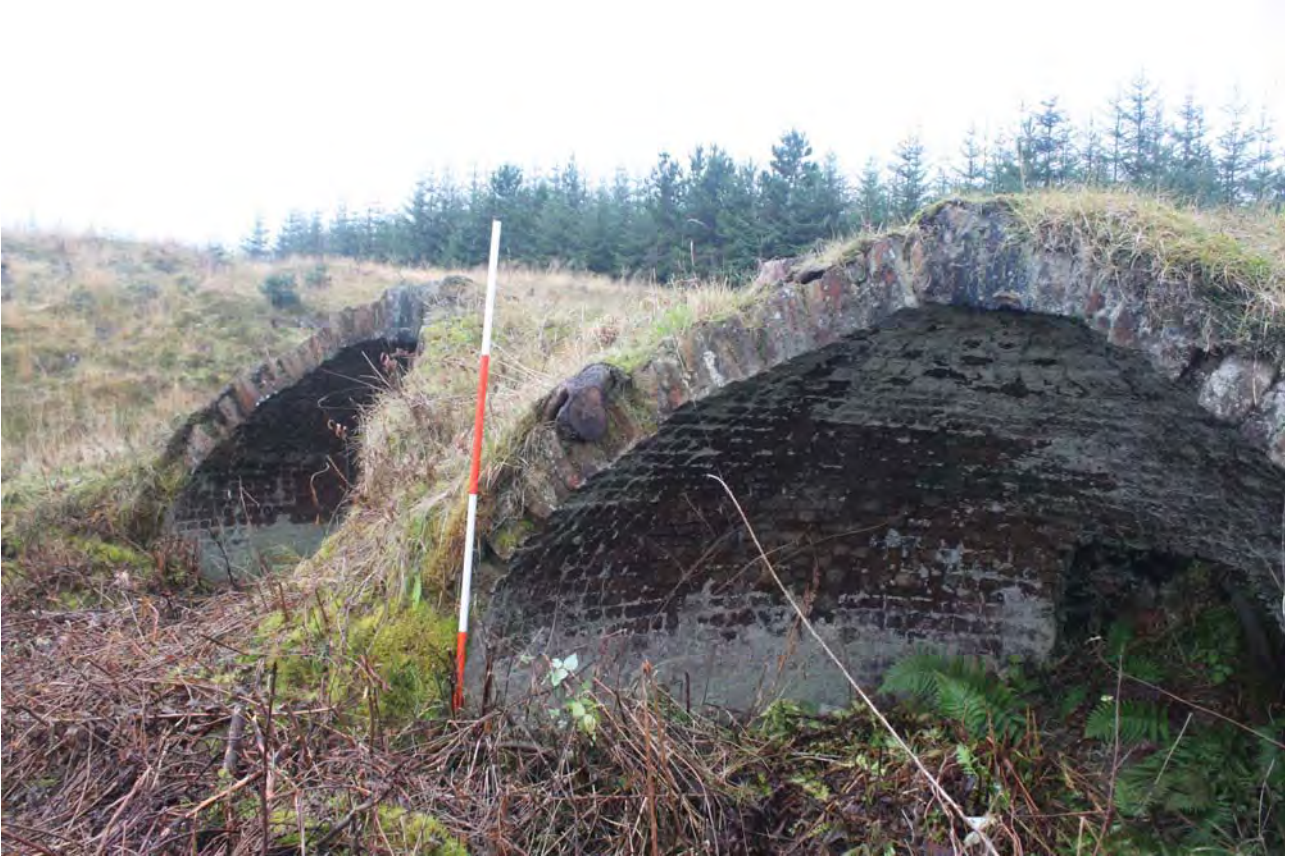
Plate 5: General view of C2 from the north-west
