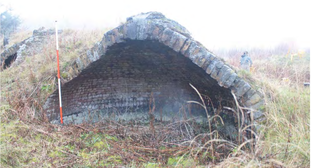
Plate 12: General view of C9 from the south
