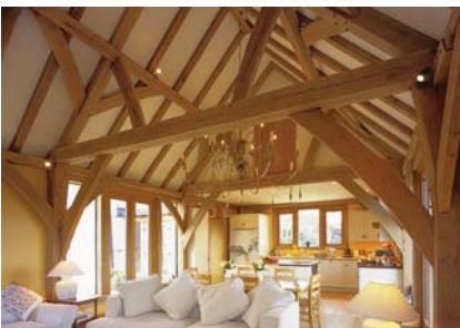
Figure 5.2 Approach A Frylands Cottage- A green oak building in traditional vernacular style and scale, framed with traditional pegged joints. Photo: The Green Oak Carpentry Company
