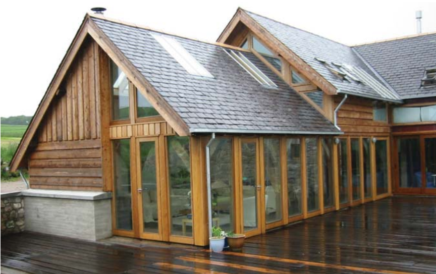
Figure 9.3.4 Exterior view of the new wing; the oak frame is enclosed within the building Photo: Bl@st Architects
