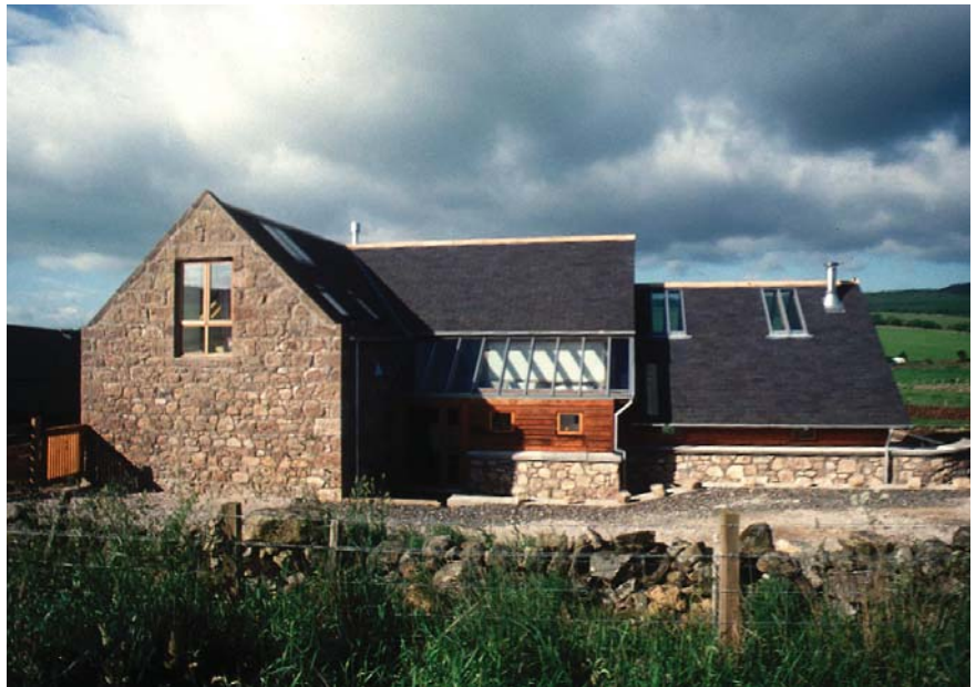
Figure 9.3 1 External view showing the original barn and new wing Photo: BI@st Architects
