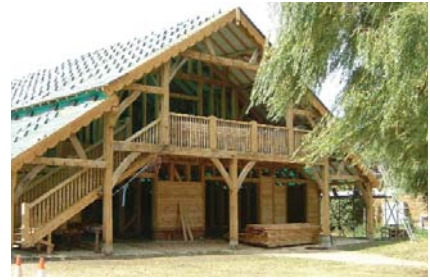
9.4 Abingdon School boathouse
