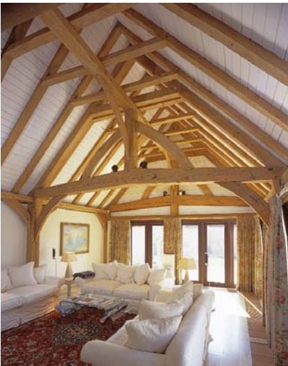
top: One and a half storeys using a modern two-tier cruck frame centre: One and a half storeys with gallery; principal frames use raking struts from the tie beam bottom: a simple crown post roof
