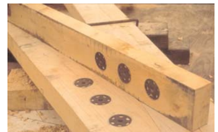
Figure 9.5.5 The scissor straps before assembly, showing the double shear connectors which will eventually be back-to-back on the same bolt. The connectors move with the timber they are set into, and do not lose strength if the timbers distort while drying Photo: P Ross
