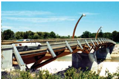
Figure 8.16 In Crest, Drôme, France, a modern bridge superstructure made exclusively from locally-grown timbers. Capable of pedestrian, equestrian and light vehicular traffic, of 33 m main span (total length 92 m). A timber bridge was created, following the demands of the town residents and others employed locally, who called for a sustainable solution, which supports their local economy Photo: C J Mettem
