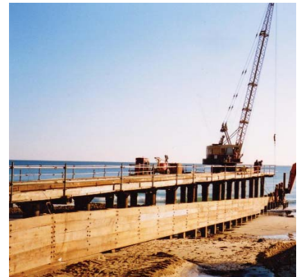
Figure 3.3 Sea defences being constructed using greenheart
