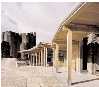
Figure 5.6 Caerphilly Castle Visitor Centre. The prominent cantilevers of the canopy are a case where special care was taken to control the vertical deflections of green oak beams. This included prediction of creep using the Eurocode methods Photo: Davies Sutton Architects
