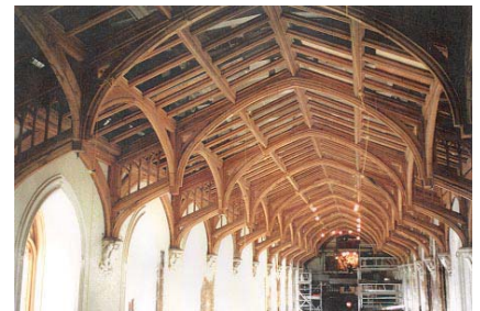
Figure 2.12 'Downsian gothic' trusses at St George's Hall, Windsor Photo: Giles Downes, Siddell Gibson Architects
