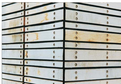
Figure 8.12 Mitred corner in green oak cladding at the Earth Centre employs a gap between the ends of the boards to disguise movement between the faces and to conceal the exposed end grain of the boards
