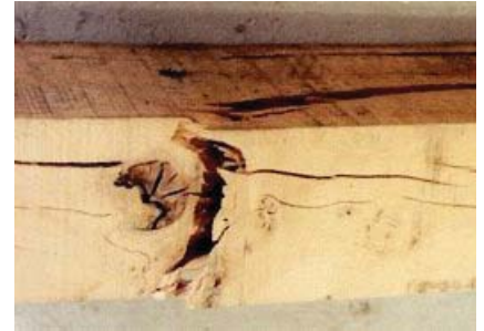
Figure 6.9 Part of an oak beam that has fractured at the end of a full-sized bending strength test. The knot on the lower surface (in the foreground - a zone of the beam experiencing large tensile strains) dictated the ultimate bending strength of the piece - a “Grade B” beam, according to the grading rules. The knot emerges from within the section, rather than being a superficial feature, and so it would be assessed carefully by the grader. In general, such knots have a more severe influence on strength than the centreknot type in Figure 6.17
