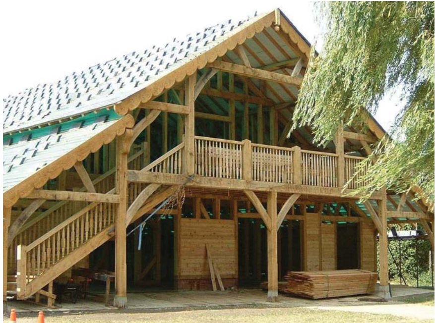
Figure 9.4.1. The completed frame Photo: Marc Nurton, Abingdon School
