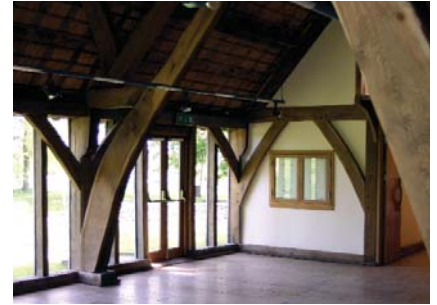
Figure 6.2 The Great Oak Hall, built in 2000 at Westonbirt Arboretum. The traditional design includes two cruck frames Photo: C Mettem
