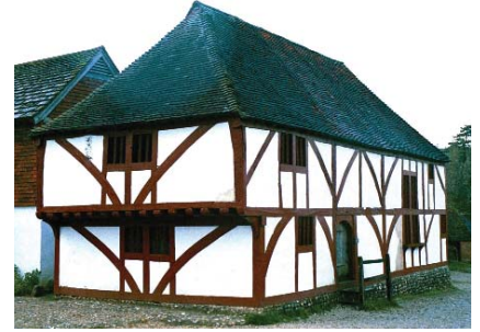
Figure 6.23 Building finished with a red ochre limewash at the Weald and Downland Museum Photo: C J Mettem
