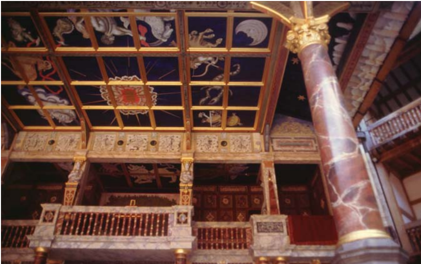
Figure 9.1.8 One of the two stage columns, looking up at the 'heavens'. They are painted to resemble marble and topped with elaborate Corinthian capitals. The stage as a whole, literally the focus of the theatre, is a riot of 'early Renaissance' decoration Photo: P Ross
