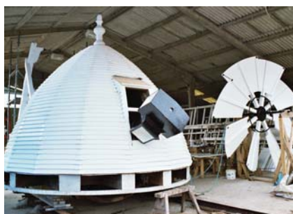
Figure 6.22 A mill cap finished with linseed oil paint Photo: C Mettem
