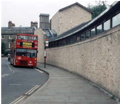
Figure 9.7.1 The Silver Street elevation with a wall of reclaimed bricks set in lime mortar. The lantern ventilator can be seen in the distance Photo: P Ross
