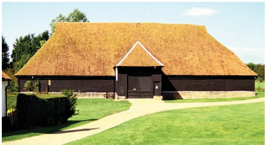
Figure 6.1 For the principal posts of buildings such as the Barley Barn, Cressing Temple, Essex (above right and left), there was a need for exceptional oaks. Extensively researched, the structure dates from 1205 – 1230 AD. At the same site, the Wheat Barn (right) dates from 1257 – 1280; hence these two buildings are amongst the oldest carpentered oak frames still in use in the British Isles Photos: Barley Barn: © Cressing Temple, part of Essex County Council Wheat Barn: C J Mettem
