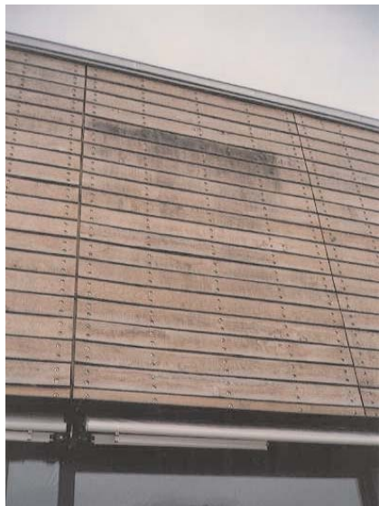
Figure 4.12 Tannin exudation on European oak cladding boards
