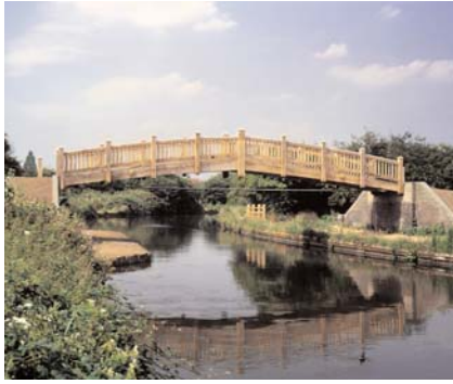
Figure 8.4 Green oak bridge for the Grand Union Canal, in Ealing, by The Green Oak Carpentry Company Photo: Green Oak Carpentry Company
