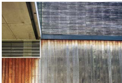
Figure 6.21 The River and Rowing Museum at Henley on Thames, built in 1996 was one of the first projects in the UK to use green oak cladding. It illustrates how small changes in exposure can produce large variations in colour Photo: P Ross
