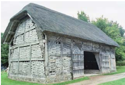
Figure 2.2 Cruck framing above and centre: Midlands cruck barn, now at Avoncroft Museum right: The Red Lion, Weobley Photos C J Mettem
