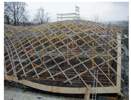
Figure 9.8.5 A timber ring beam provides the boundary to the gridshell structure Photo: Buro Happold / Weald and Downland Museum
