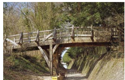
9.11 Polesden Lacey bridge
