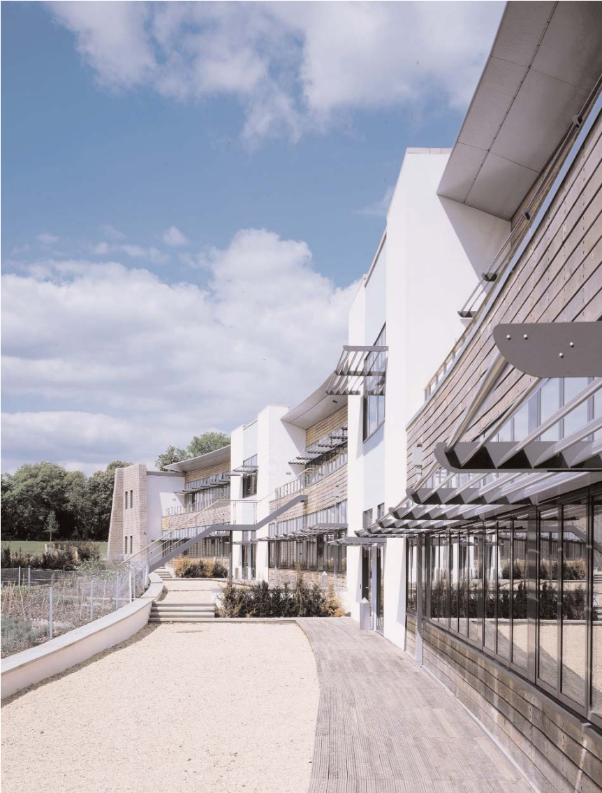
Figure 8.14 Green oak decking and cladding is a feature of this office building Photo: Brocklehurst Architects
