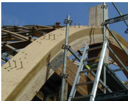
Figure 9.8.7 At the entrance the shell connects to a European larch glulam arch Photo: Buro Happold / Weald and Downland Museum
