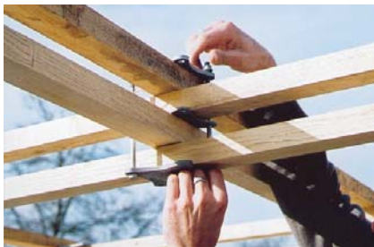
Figure 9.8.6 The node connections utilise a patented system of steel plates and bolts. The connector comprises three steel plates, with the central unit having pins to locate grid layers 2 and 3, whilst the outer plates loosely hold layers 1 and 4 until clamping occurs. Two of the four locating bolts also connect the diagonal braces Photo: Buro Happold / Weald and Downland Museum
