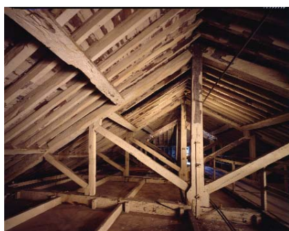
Figure 2.8 King post truss. Roof of Trinity College, Cambridge. Photo: Jewell Harrison
