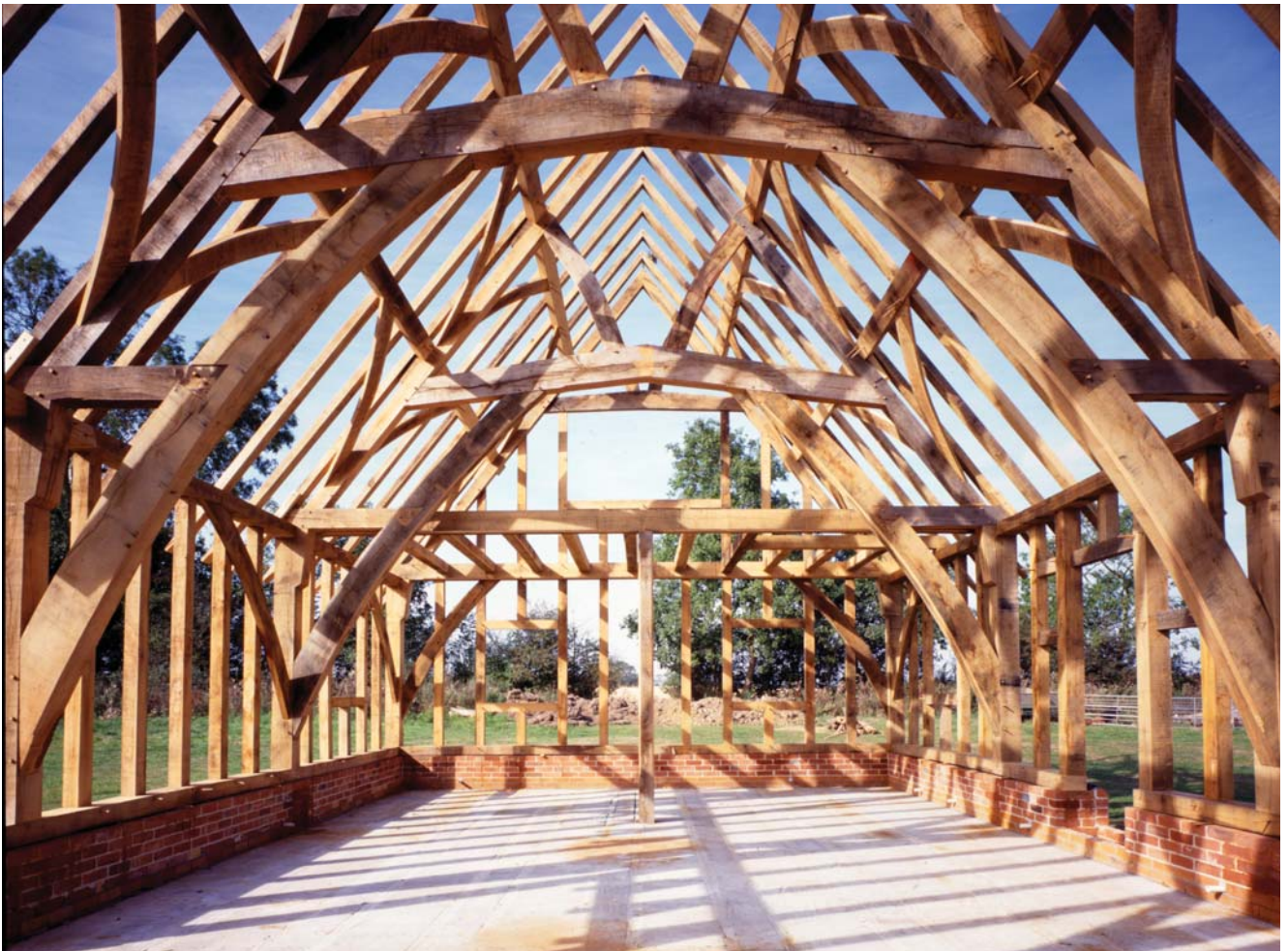
Figure 2.10 (and next page) Modern green oak structures Framing and photos: The Green Oak Carpentry Company below: Completed frame before enclosure
