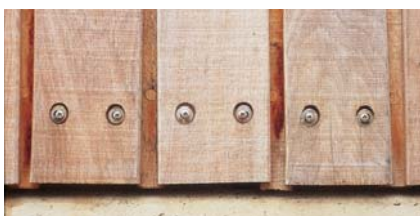
Figure 8.13 Use of oversize washers to allow movement in green oak cladding Photo: P Ross
