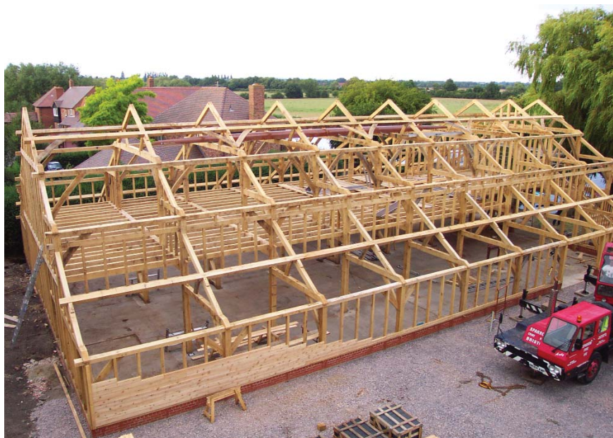
Figure 9.4.8 The bare frame nearing completion Photo: Ginette Guiver
