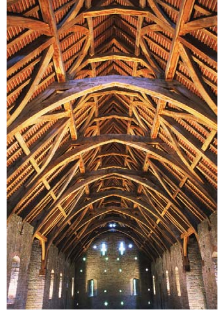
Figure 2.11 (above and left) Pilton Barn, Glastonbury. Reconstruction of roof destroyed by lightning Framing: McCurdy & Co Architect: Caroe and Partners Photos: Wood Awards / McCurdy & Co
