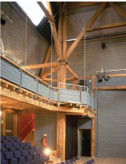
Figure 9.6.3 Balcony support Photo: P Ross
