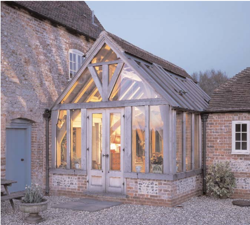
Figure 8.3 A small modern green oak frame having sill beams mounted on a low brick and flint wall. The detailing also avoids the commonly-found problem with older buildings of decay at the base of the door posts, another position at which there used to be water uptake through end grain
