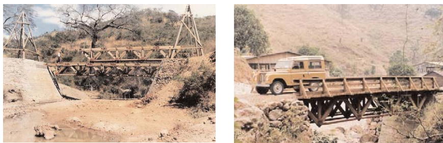
Figure 8.22 Modern system-built light vehicular bridge, widely used in several world regions. Suitable for incorporation of strength graded air-dried European oak Photos: C J Mettem
