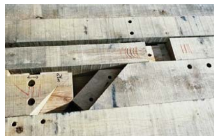
Figure 1.2 Prefabricated sections of green oak framing ready for delivery to site Photo: C J Mettem
