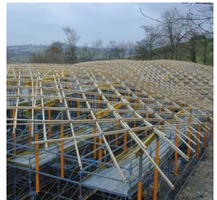
Figure 9.8.4 The double layer grid partially lowered into place Photo: Buro Happold / Weald and Downland Museum
