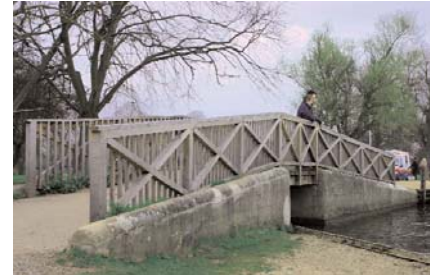
Figure 8.17 A typical oak footbridge of modest scale on the Thames towpath, at Marlow, Buckinghamshire. The parapet design reflects a famous nineteenth century suspension bridge crossing the river nearby Photo: C J Mettem
