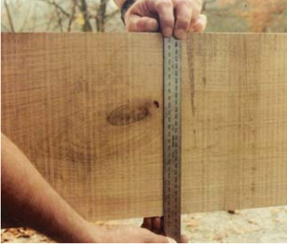
Figure 6.6 Measuring the external surfaces of knots and estimating their internal location and influence is one of the most important tasks in visual strength grading. The oval knot near the centre of the beam is a feature common in oak, and is specifically addressed in the rules
